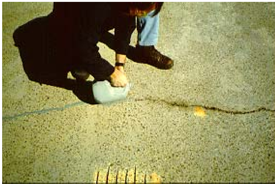
Figure 5. Applying Modified Grout to Seal RMP Crack.
